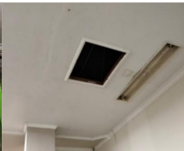
Figure 5. Condition of lighting
